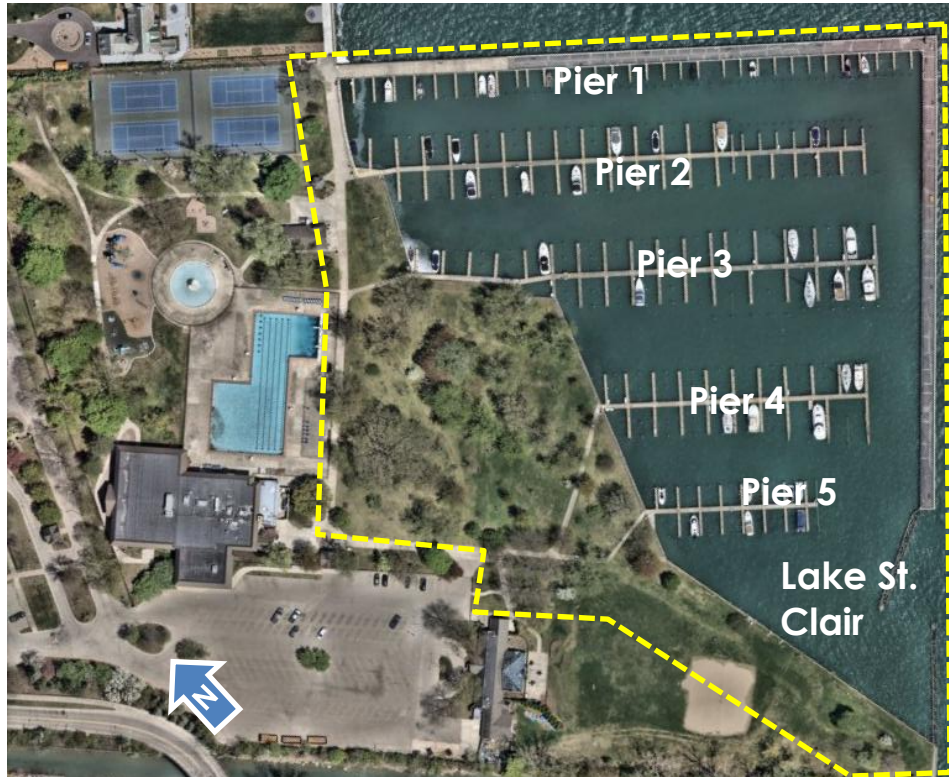
Figure 1: Nearmap aerial image (4/30/2025) of GPP WPP Marina
