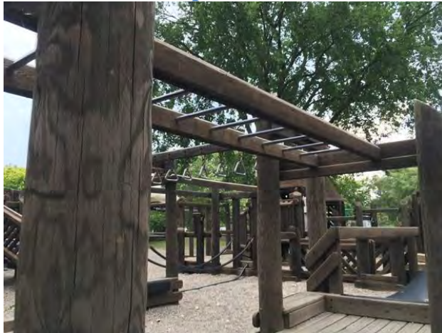
Horizontal Ladder picture #1
