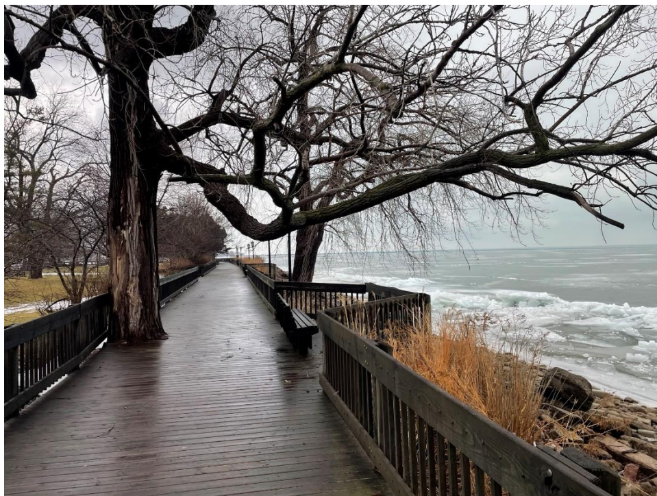
Figure 5 - Location along boardwalk with slipping hazards and low clearance (6'-8'')
