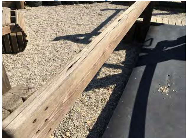
Rubber bridge 5-12 area picture #2
