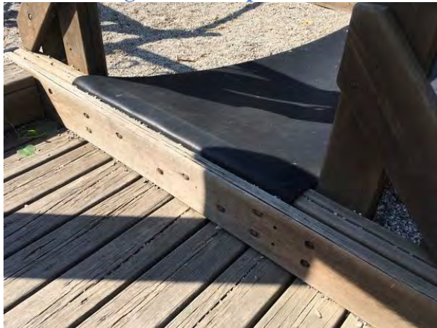
Rubber bridge 5-12 area picture #1
