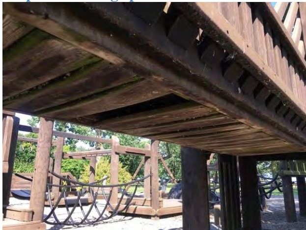
Suspension bridge picture #1
