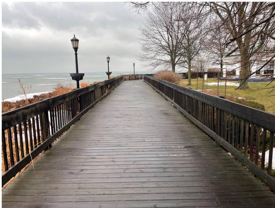
Figure 1 - Typical view of boardwalk structure - looking southeast
