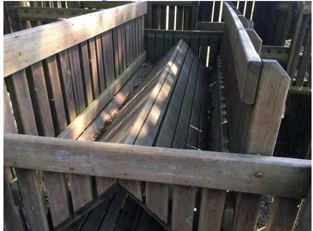
Crawl Tunnel picture #2
