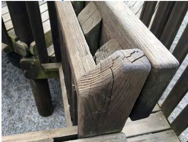
Handrail post picture #1
