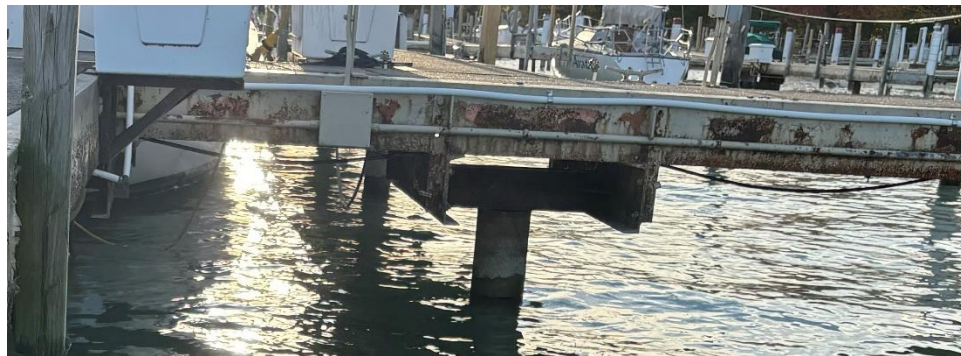
Figure 14: Typical main pile connection at Piers 3 and 4.
