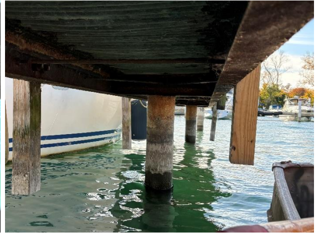
Figure 16: Typical finger pier pile connection.
