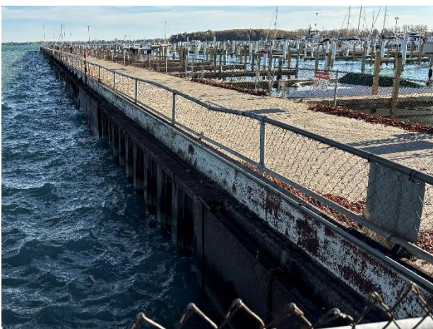
Figure 29: East breakwall, north end.
