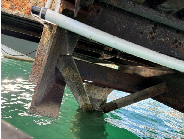
Figure 18: Reinforced pile connection (Pier 4). Figure 19: Shimmed pile connection (Pier 3).
