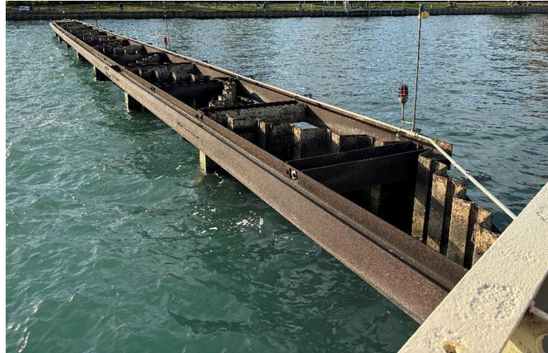
Figure 28: East entry wall.
