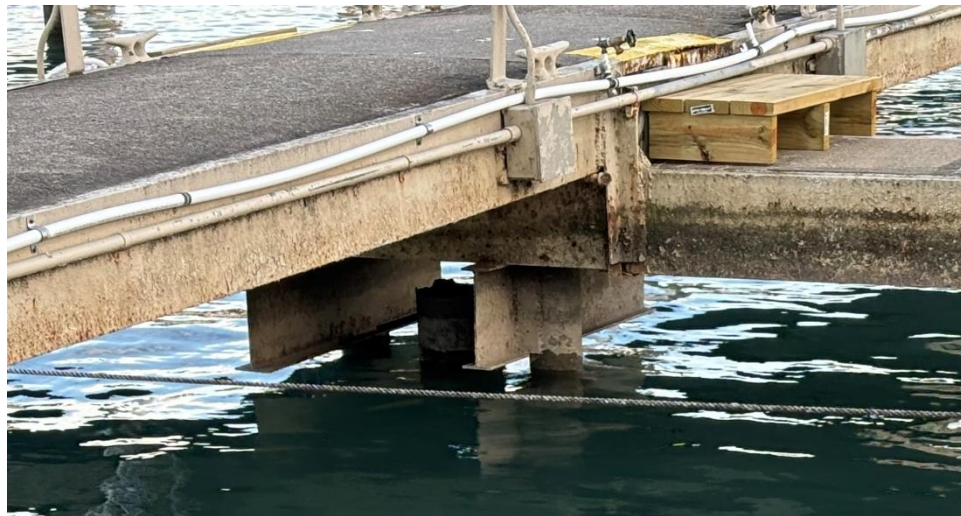
Figure 20: Abandoned pile with two new piles to support pier (Pier 2).
