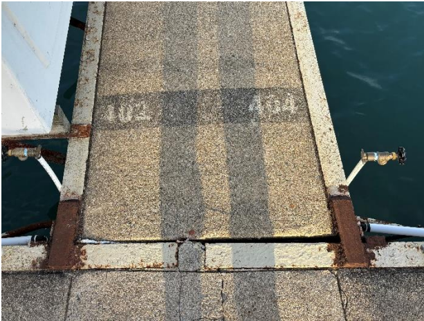
Figure 10: Frame joint reinforcing on Pier 4.
