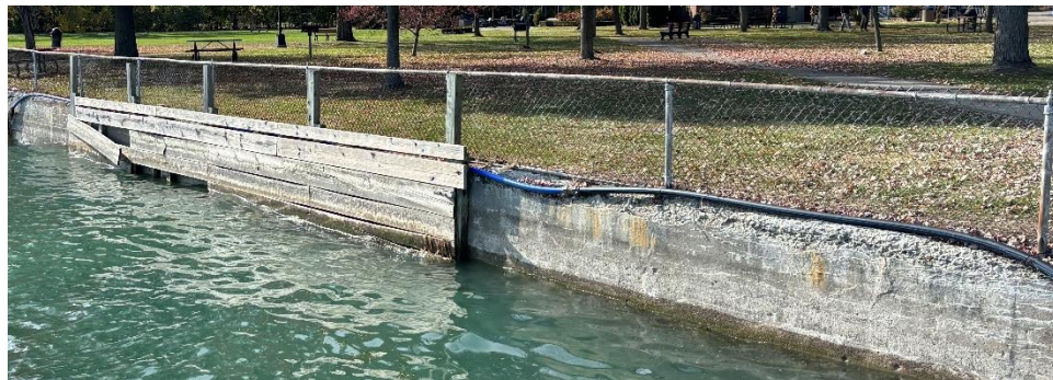
Figure 23: North concrete seawall between Piers 4 and 5.
