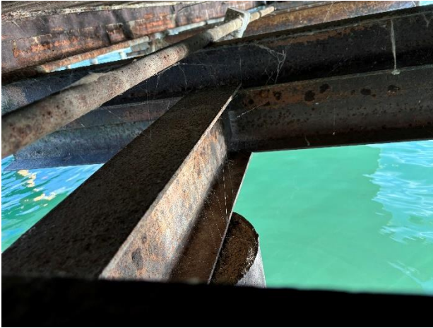
Figure 15: Typical main pile connection.
