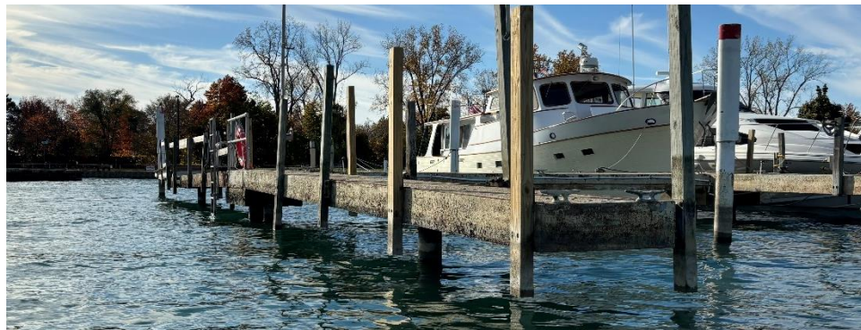
Figure 32: End of Pier 4.
