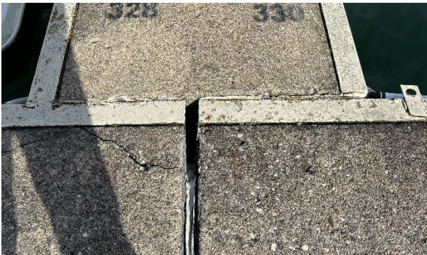
Figure 8: Widening deck joint on Pier 3.
