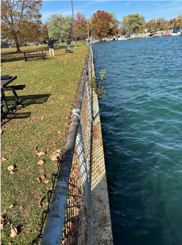
Figure 24: West seawall, looking North.
