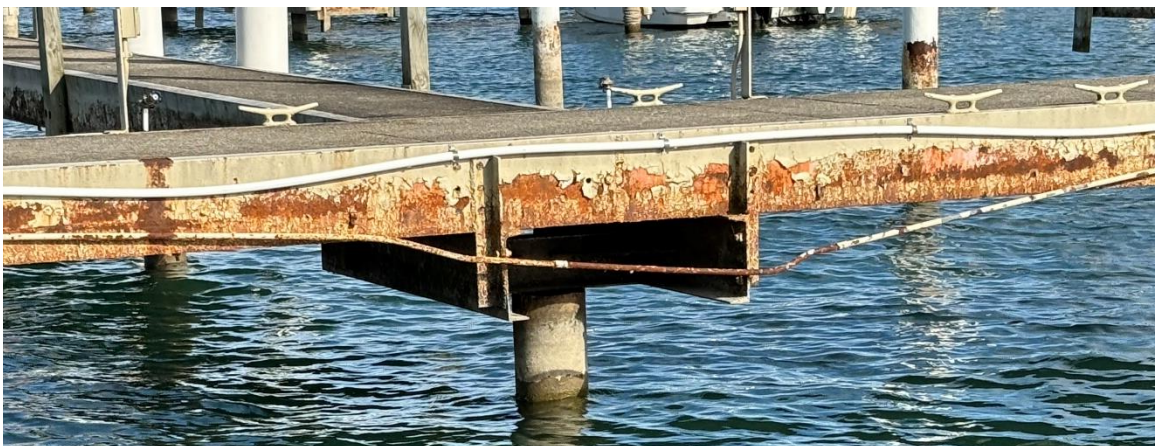
Figure 12: Typical condition of steel pier frame.
