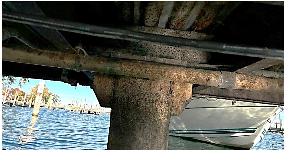
Figure 17: Typical main pile connection at Pier 5.
