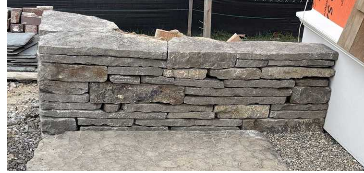
DRY STACKED STONE RETAINING WALL
