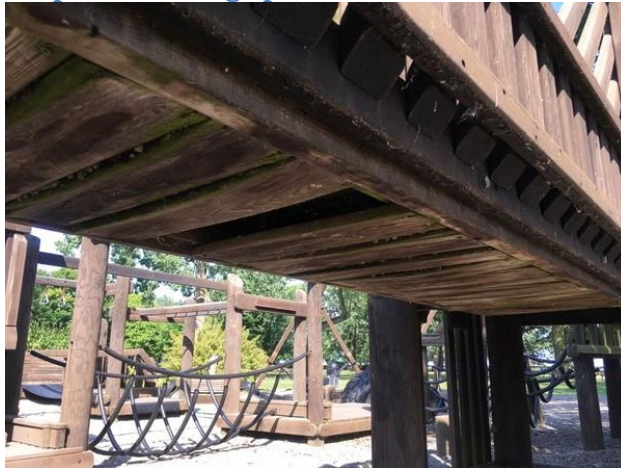
Suspension bridge picture #1
