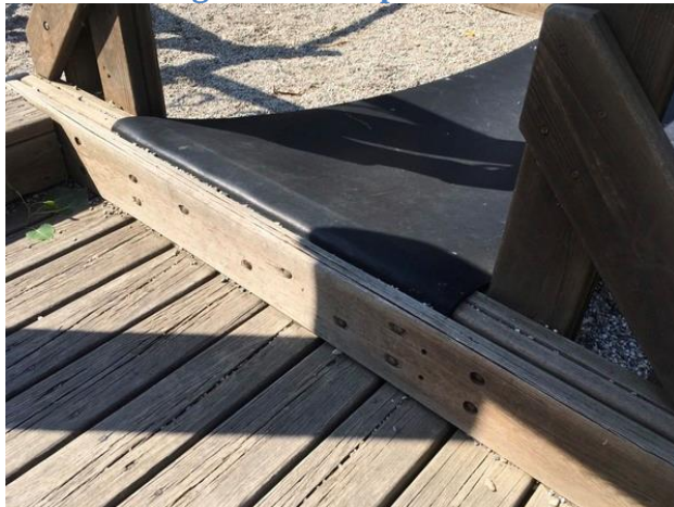
Rubber bridge 5-12 area picture #1
