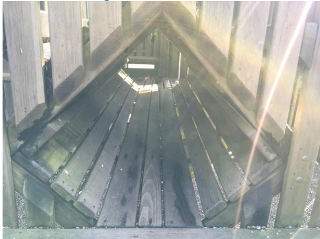
Crawl Tunnel picture #1
