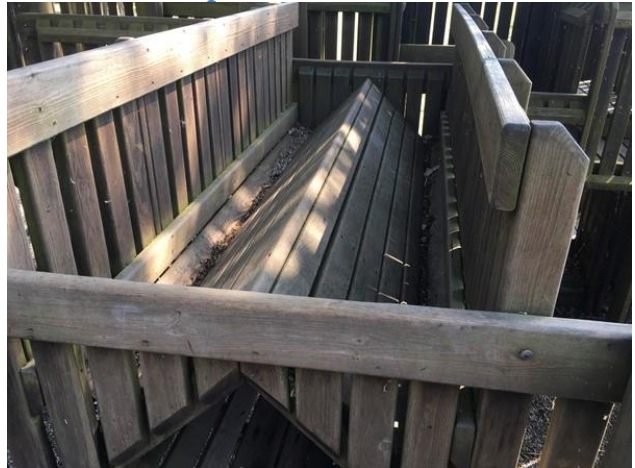
Crawl Tunnel picture #2
