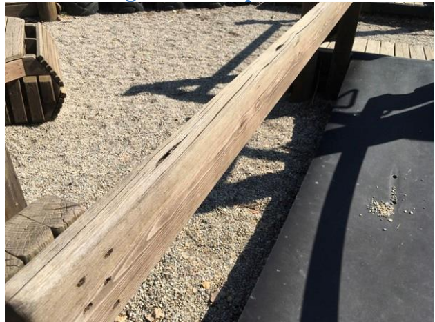
Rubber bridge 5-12 area picture #2
