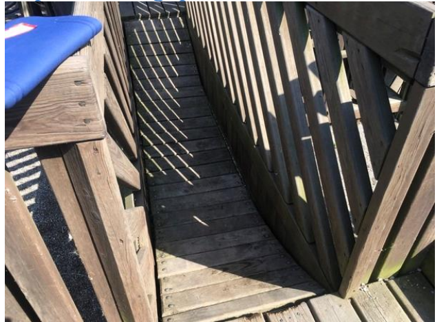
Suspension bridge picture #2
