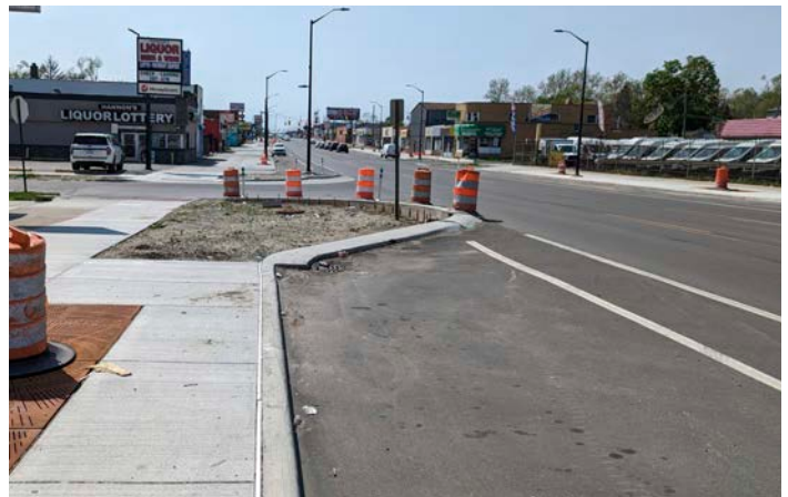
West Warren, ongoing construction, summer 2023
